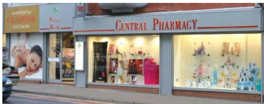
Central Pharmacy is immaculate from top to bottom – from the well-appointed offices on the top floor, to the pristine street frontage.
